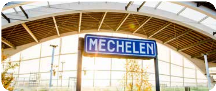
Project nieuw station Mechelen
