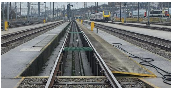
Figure 69 : Fosse de visite
